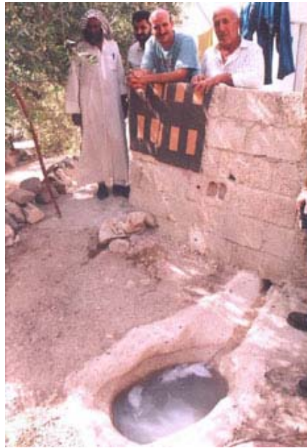
Figure 4.1: Graywater storage in Adasiyyah (Photograph by CSBE)
