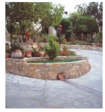
Figure 25: Paved areas directed to catch rainwater via a small collection channel.
