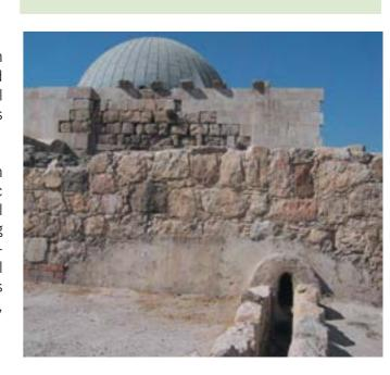
Figure 21: A historical example of water harvesting at the Amman Citadel. Water collected from the roof is directed through channels toward water storage areas.
