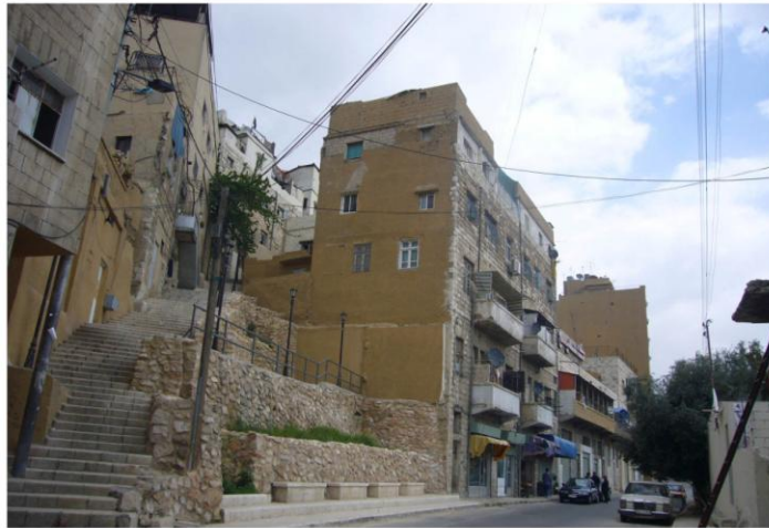
Figure 12a: Painting concrete facades in Jabal al-Qal'a
