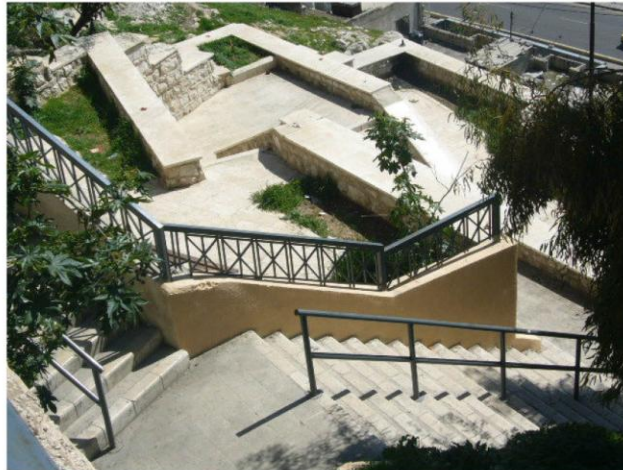
Figure 3c: Stairway leading to Raghadan Complex
